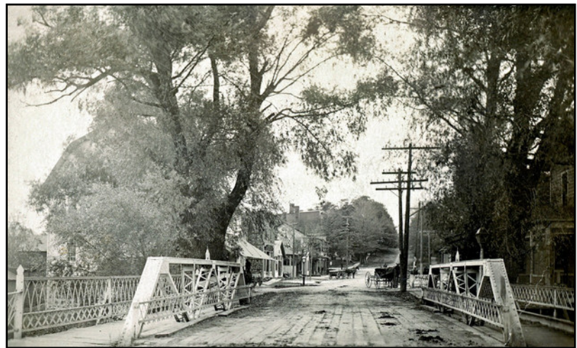
Looking east on Main St. in Gorham
